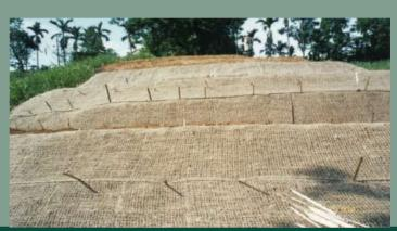
Jute Geotextile (JGT) is a fabric made from 100% jute fibre. Different types of JGTs have been designed and developed for use in the geotechnical field of applications. The products have been standardized by BIS and also included in the Schedule of Rates by WBSRDA, PWD (Roads) Govt of WB, Govt. of Assam, Govt. of Meghalaya, R&B department Govt. of Gujarat, BRO, Irrigation & Waterways, Raliways etc. IRC has also published guideines (IRC SP 126-2019) for road construction with the use of JGT.
